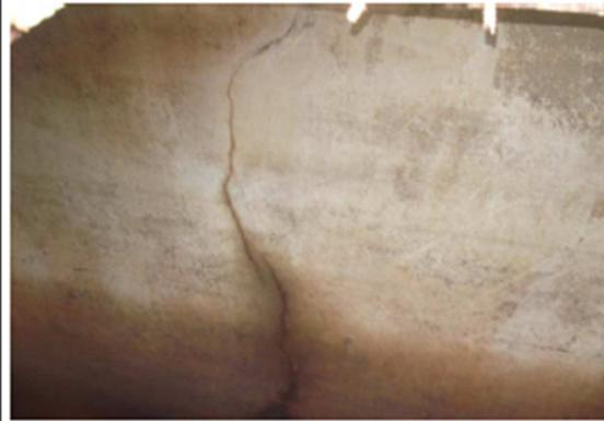
VISTA INTERIOR DONDE SE APRECIA LA GRIETA EN EL TANQUE.
