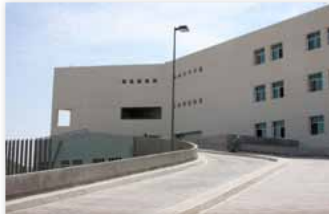
Hospital Regional General del IMSS
