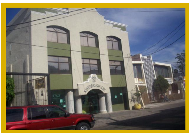
HOSPITAL SAN JOSE
